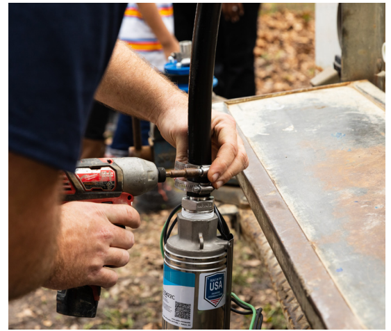
A member of the Creason Well Service team is preparing to install the new well pump.
