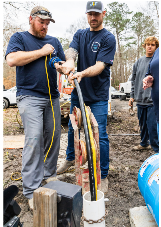
Chris Long assisting members of the Creason Well Service team with installing the new well pump.
