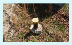
What is Proper Permanent Well Abandonment? Permanent Well abandonment is not simply capping the well as shown in the photo to the left. Capping the well is only considered to be temporary abandonment. Permanent abandonment involves completely filling the well with grout as described in the steps below.
